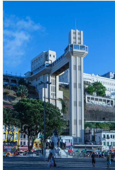
(b) Elevador Lacerda, built 1869–1873, then the world's highest elevator. Public domain.
